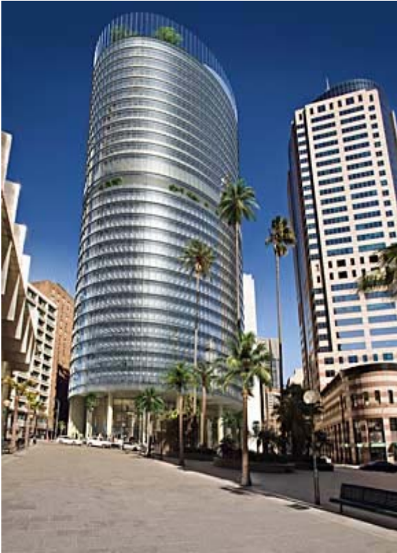
Sydney’s new Six-Star Green Star Office Building at 1 Bligh Street.
